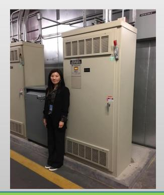
In this picture a Variable Frequency Drive powering a Main Terminal Air Handling Unit fan running at 350 Horsepower
